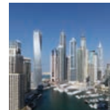
DUBAI Saving energy in air conditioning systems
